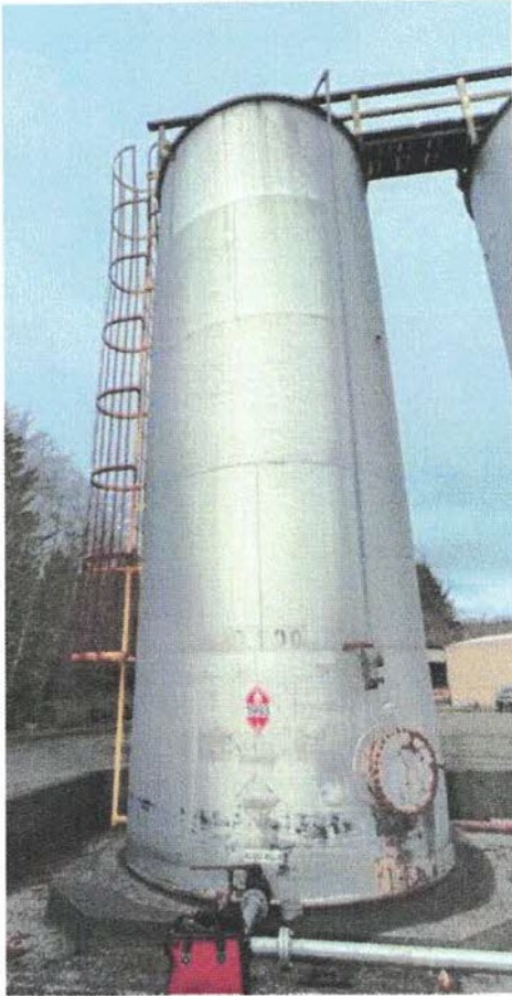
Figure 3 - Aboveground Storage Tank from CX 04
