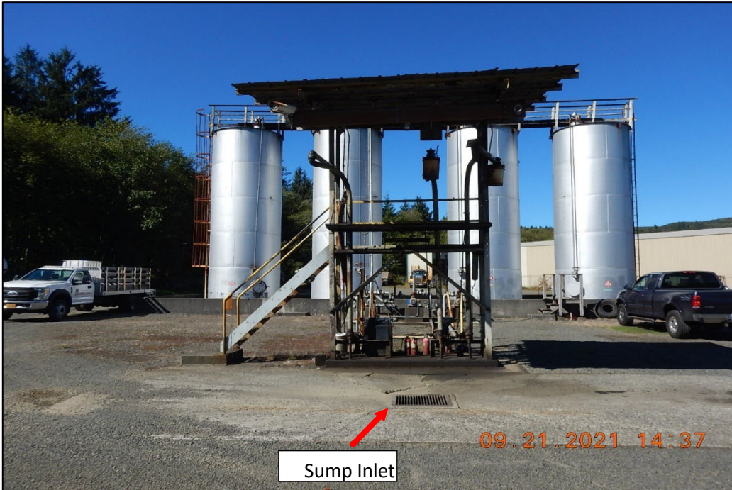
Figure 2 - Four Aboveground Storage Tanks Within Secondary Containment
